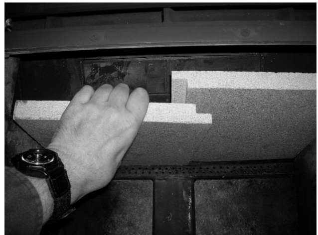
Figure 18 - Removing/Replacing the Baffle for Inspection
